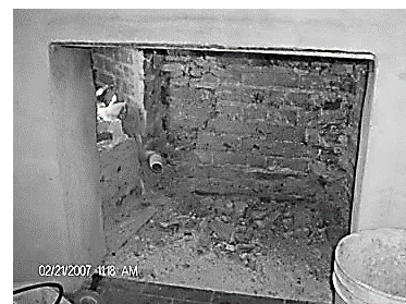
Badly Deteriorated Firebox
