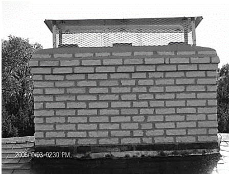
Metal Cap on Clay Liner Chimney Top
