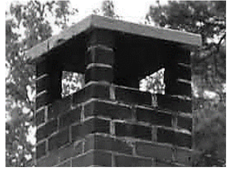
Concrete Cap Chimney Top
