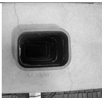
Clay Tile Liner Flue
